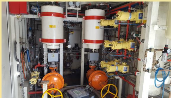
Steel shot injection system
