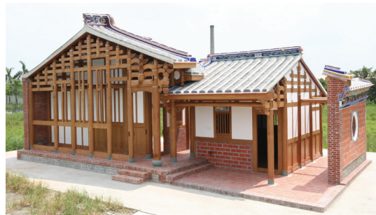
Image 25. The Techniques Reconstruction Zone (Tinghsin Hote Foundation).
