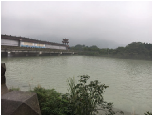
Image 5. Feishayan Spillway (Mikiko Ishikawa).
