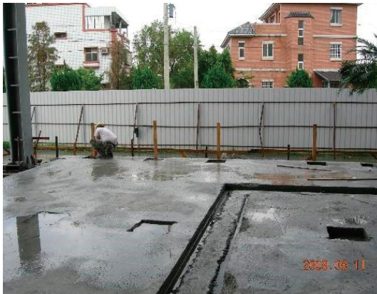
Image 20 and 21. The new raised foundation leaves space for future piping/electricity systems (Tingshin Hote Foundation).
