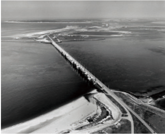
Image 7. The Oosterscheldekering is part of the Delta Works. The Oosterscheldekering has slider barriers that are only lowered at high tide. In normal situations, when the gates are open, the natural tidal dynamics are left undisturbed (Source: Beeldbank RCE).
