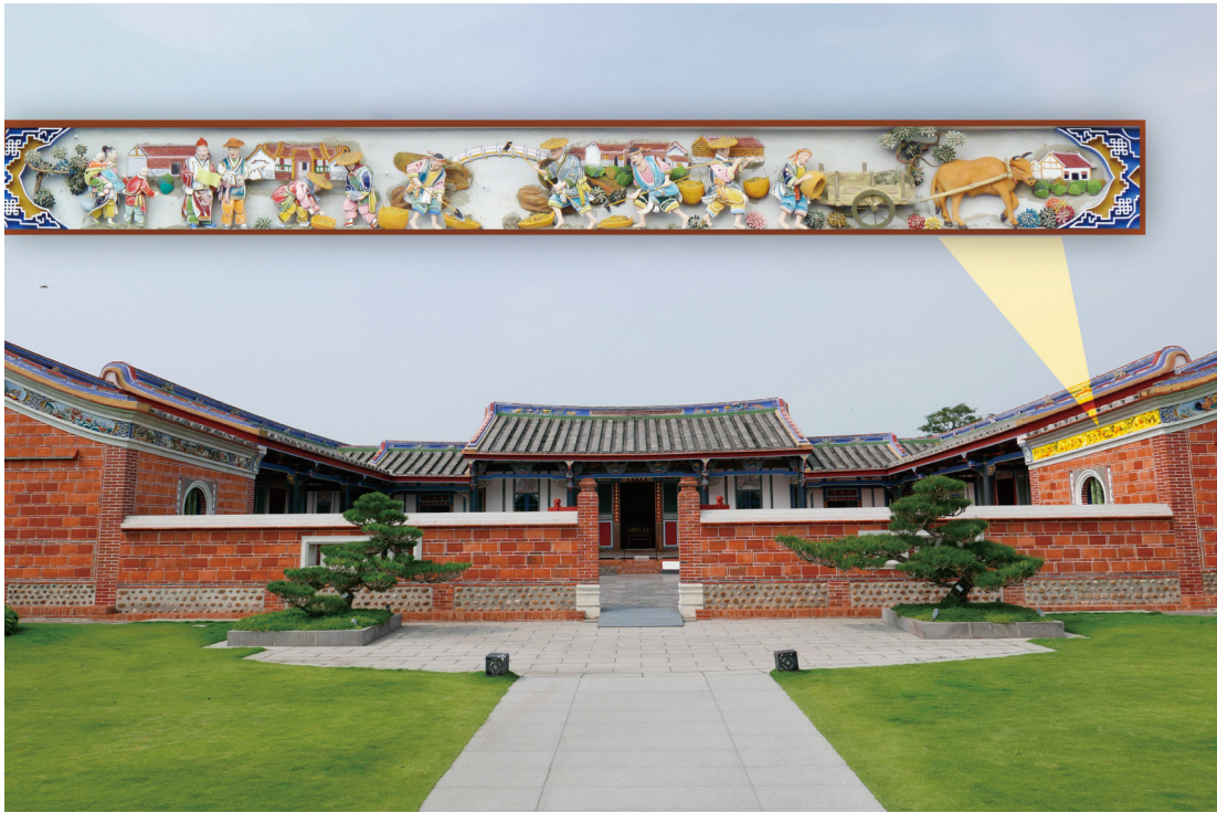
Image 29. The ceramics cutting and pasting decoration on the cornice depicting the scene of the Wei family's contribution to the Babao Canal (Lin, 2019).
