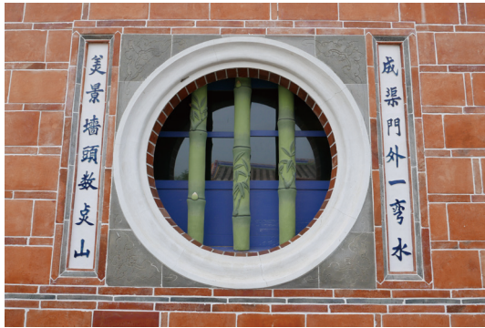
Image 30. The couplets on the sides starting with the characters ‘成’ (cheng) and ‘美’ (mei) indicate the estate’s inseparable relation with the Second Babao Canal.
