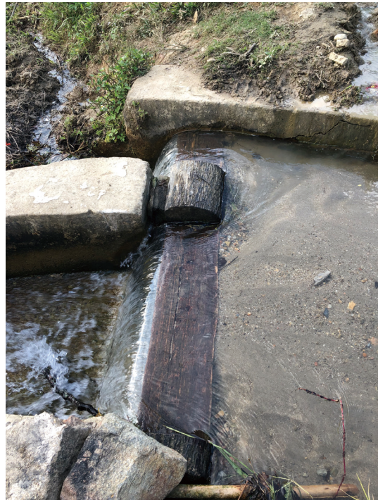
Image 6. Historic Wood cut system for water sharing at Honghe Hani Rice terraces in China (Nupur Prothi Khanna).
