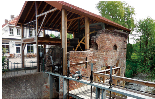
Image 14. The St Elisabethsmolen in Haelen has partly been rebuilt in 2015 and now has a turbine which produces 50,000 kWh/year. The electricity is used by the next door restaurant (SLL).
