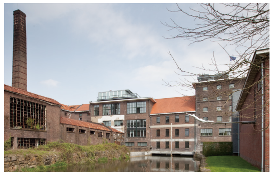
Image 16. The ECI hydroelectric power station (RCE, K.Roderburg) is the only remaining watermill along the Roer and Vlootbeek streams. The turbine's output is 250 kWe. However, owing to the lack of water, this will rarely be achieved.
