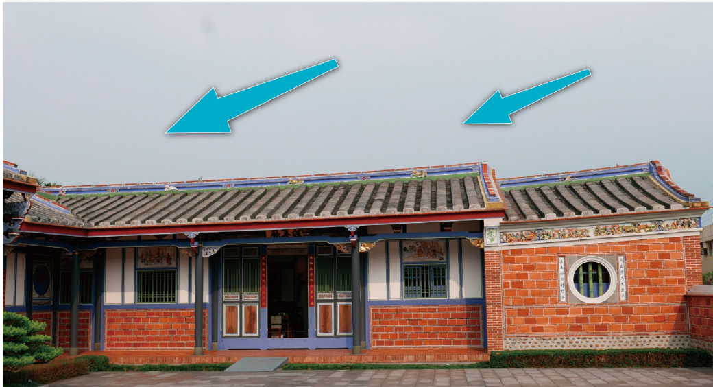
Image 12. The first room of the inner courtyard tilts and leans towards the main structure, which stands for the family’s business that relies on a secure foundation and implies ‘Keeping the wealth within the family’ (Photographed by Queenie Lin, 2019).
