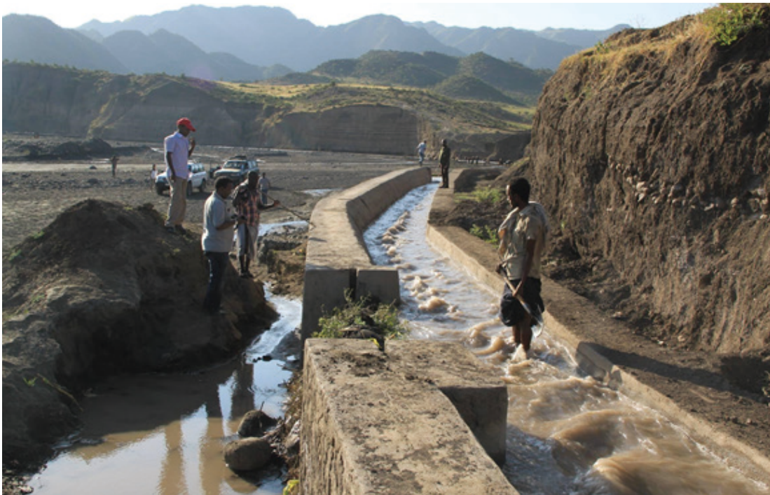
Image 2. A cemented stone masonry work canal in Ethiopia's Raya region used to divert seasonal river floods (Source: Spate Irrigation Network Ethiopia).
