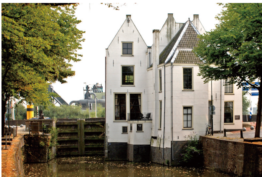
Image 4. Harbour Lock (Havensluis) (Nico Boerboom).
