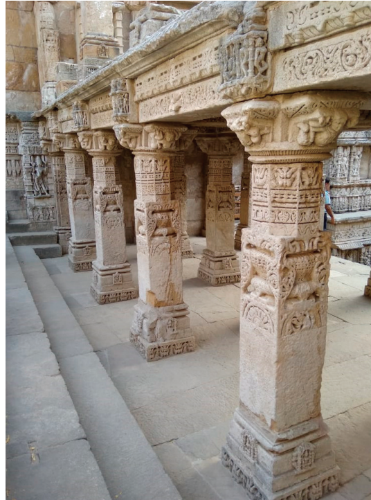
Image 3. The descending access to the well is flanked by intricately sculpted columns supporting intermediate pavilions in the Rani ni vav. Photo by Dimple Mehta.
