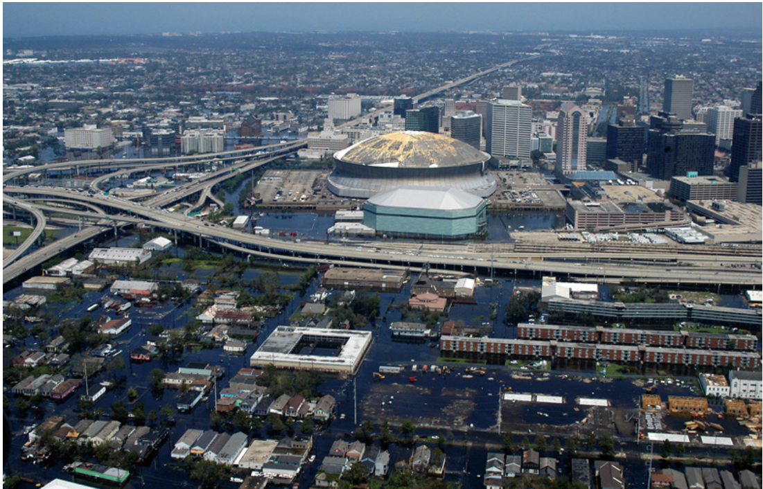
Image 8. More than fifty failures in the levees and flood walls protecting New Orleans led to extensive flooding after Hurricane Katrina in 2005 (Jeremy L. Grisham—U.S. Navy).
