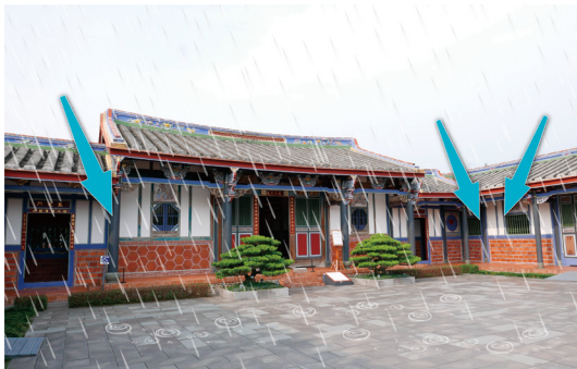
Image 13. The turning slope eaves (轉溝) which allow the rainfalls collected towards the courtyard bear both moisture adjustment function and auspicious meaning.
