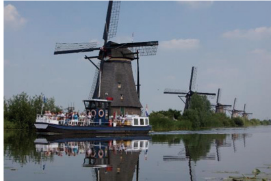
Image 4. Since the 15 th century, windmills were built to pump the water out of the polders. The nineteen monumental windmills at Kinderdijk were built around 1740. Kinderdijk was designated a UNESCO World Heritage Site in 1997 (Source: Beeldbank RCE / P. van Galen, 2010).
