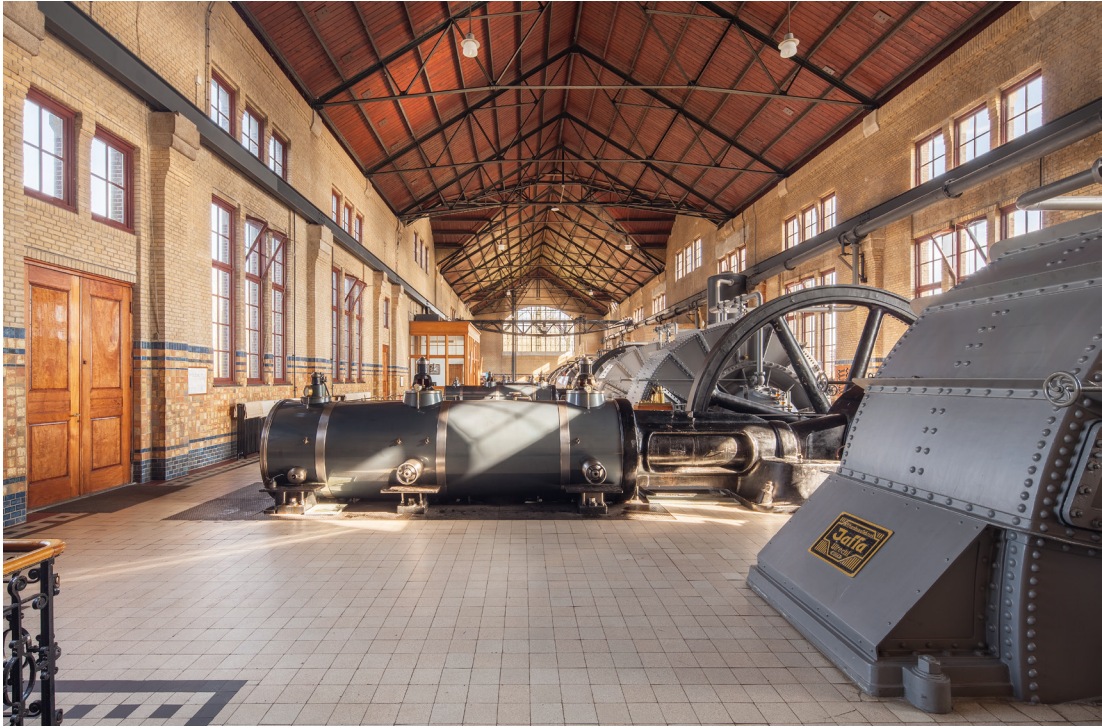
Image 2. Wouda pumping station interior (RCE, W. van der Sar).
