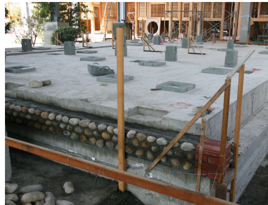
Image 20 and 21. The new raised foundation leaves space for future piping/electricity systems (Tingshin Hote Foundation).
