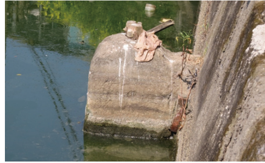
Image 8. An example of Tongharm with a removable plug.
