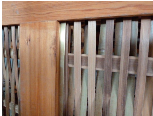
Image 27. The new water insulation mechanism installed during conservation (Tinghsin Hote Foundation).
